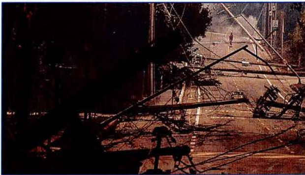
Figure B-8 - Downed power poles and lines in 2017 Tubbs Fire Photo by LA Times
